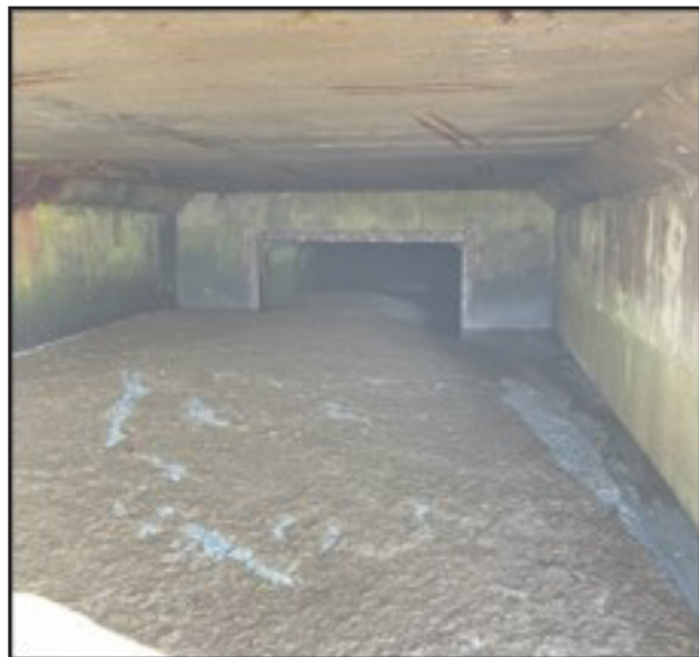
Figure 17. Sand Buildup in Lynn Outfall
