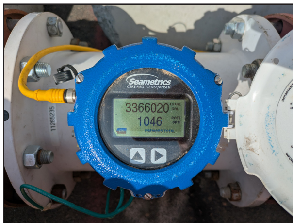
Figure 19. Flow Meter on Pump Discharge
