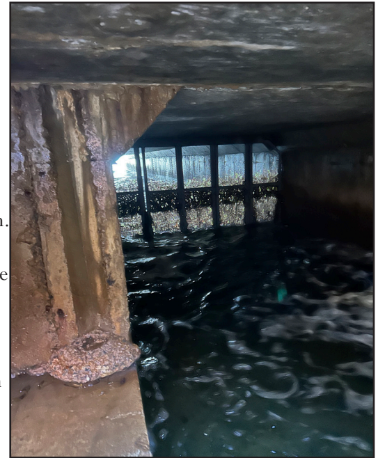
Figure 15. Culvert Screen Installed to Manage Seaweed
