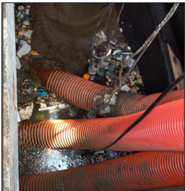
Figure 18. Wet Weather Debris in Culvert
