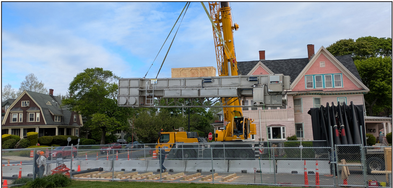
Figure 3. UV and Pumping Systems Being Installed at the Pilot Site
